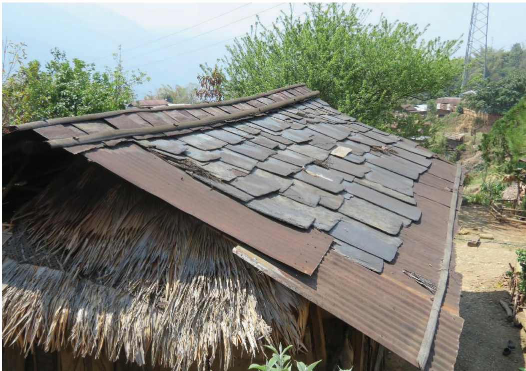
Figure 5: Traditional slate and palm thatch roofing in Old Peshu
