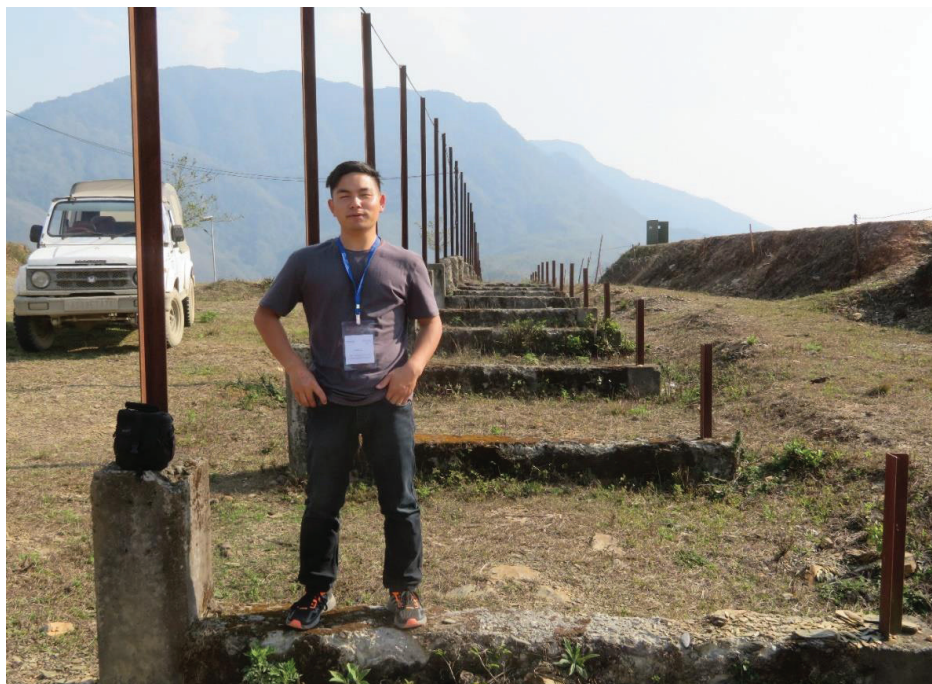
Figure 3: Abandoned border fence at Dan Village
